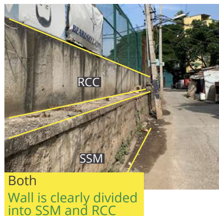
Reinforced Cement Concrete (RCC) Identified by the flat and vertical concrete slabs
