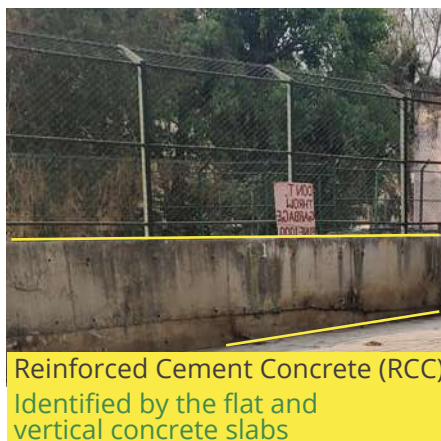
Both Wall is clearly divided into SSM and RCC
